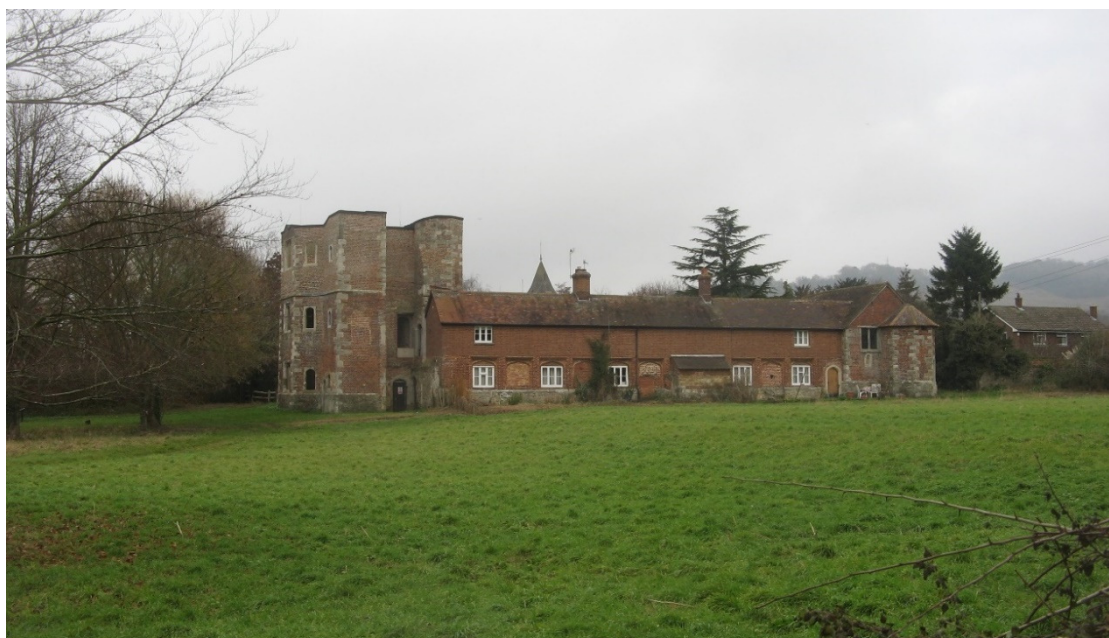
Fig 21 The north-west range seen from the south-west across Old Palace Field; note terrace marking site of former west range of outer court
