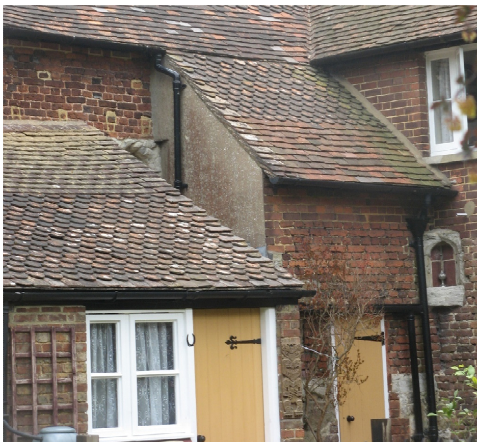
Fig 16 The remains of the added garderobe tower – the doorway is a 20 th century insertion
