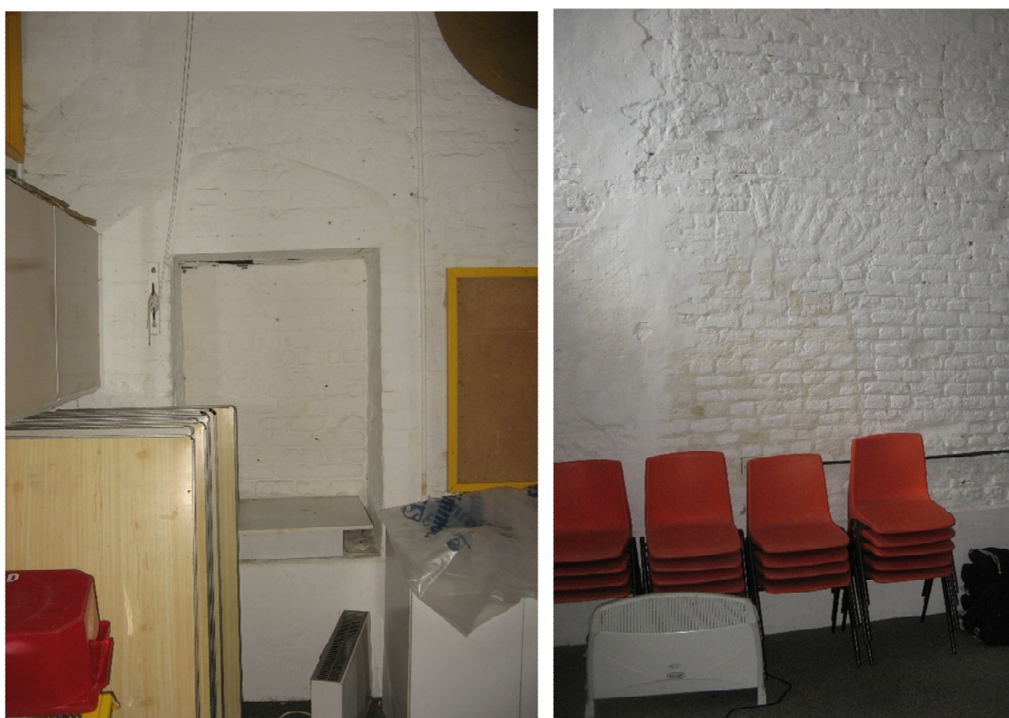
Fig 12: Gatehouse: Blocked doors from gate passage (left; for outside see fig 10) and west cloister (which appears to be secondary)
